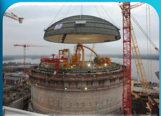
Korean NDT Companies have extensive experience in the NDT for nuclear power plant components.
